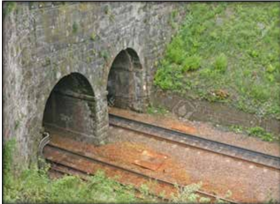
Figure 1: The Falkirk Railway Tunnel in Scotland
